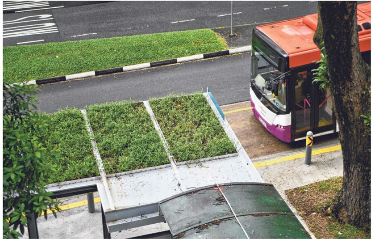
A green-roofed bus stop in Serangoon Central. As at July, about 30 bus stops have been fitted with green roofs, said a spokesman for the Land Transport Authority (LTA). Preliminary studies have shown that such roofs can lower ambient temperatures by "around 2 deg C", said LTA. ST PHOTO: ARIFFIN JAMAR
